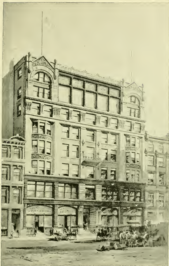
JOHN HANCOCK BUILDING.
